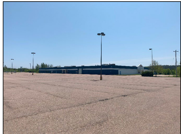
Figure 1 Former Minacs call center located at 24 Queen Street Extension.
