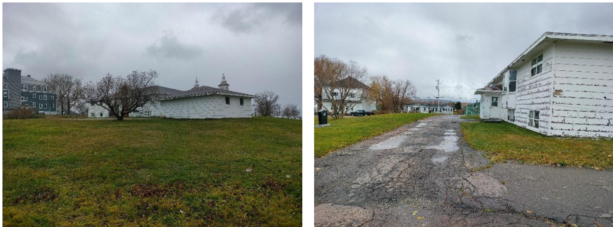
Figure 2 Images of existing site conditions
