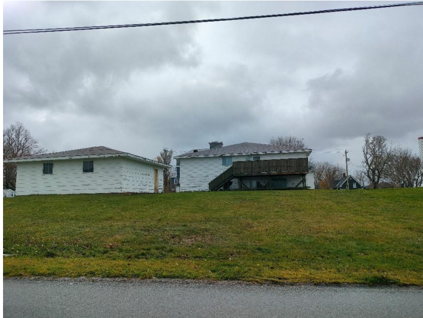
Figure 5 Image of existing buildings on the site
