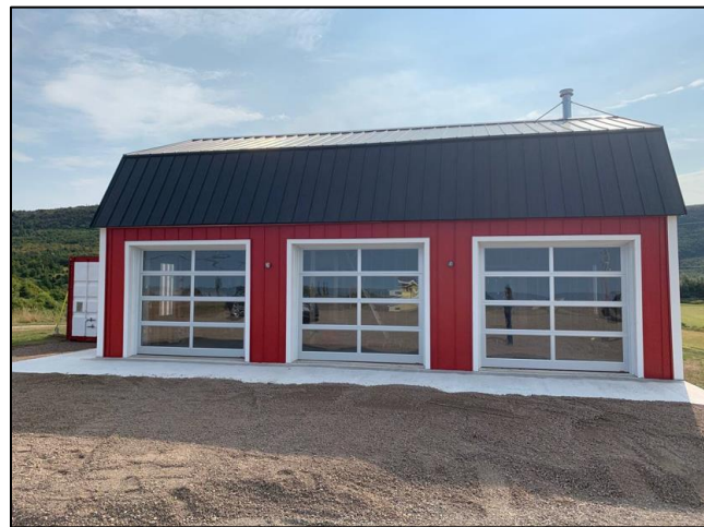
Figure 1 Existing barn to be used as a “test kitchen.”
