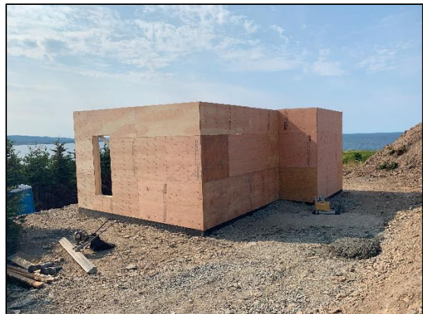
Figure 1 Rental cottage under construction, September 13, 2024.
