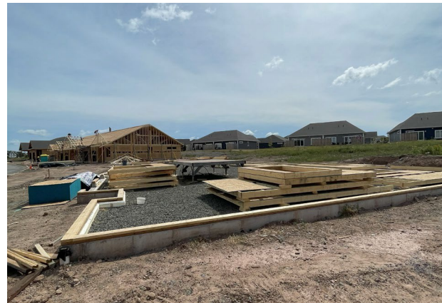
Figure 3. PID 10137099 Quadplex Foundation with PID 10137099 and PID 10137131 Framed Buildings in the background
