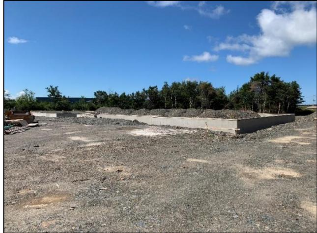
*Figure 1: Existing foundation of the 16-unit building.*
