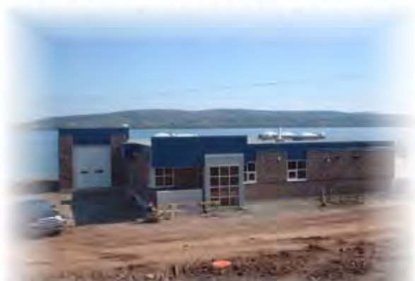
Baddeck Sewage Treatment Plant
